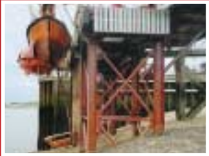
Offshore training rig supports coated with Chemi-Tech UW, a corrosion resistant lining for underwater environments.
